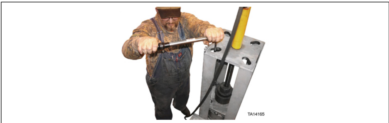
Figure 61. Installation of bolts securing inner canister components
